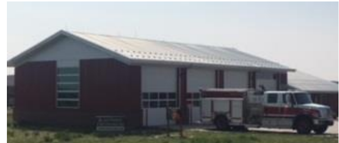
-Station #2, 16465 Ridge Run Rd.
